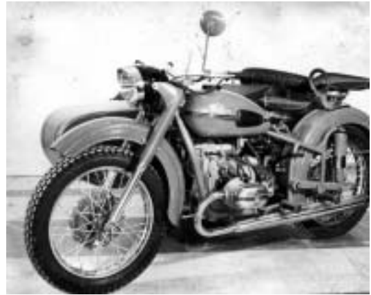
Ural M63, the first Ural to be imported commercially into England. Also note front mudguard as per M62 and introduction of the rear swinging arm.
